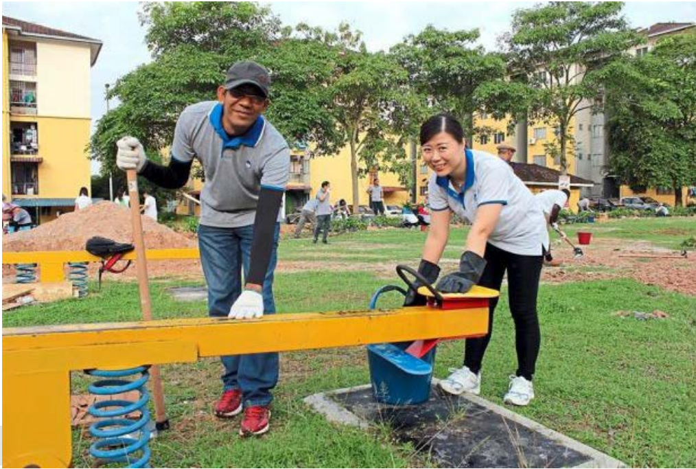
IJM employees repairing broken playground equipment.
