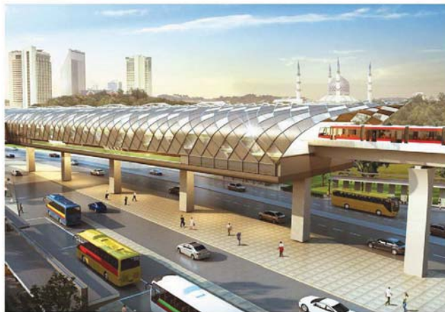
An artist impression of a light rail transit line 3 station. The contract value has boosted the group's outstanding order book to an all-time high of RM9.7 billion, IJM said in a statement yesterday.
