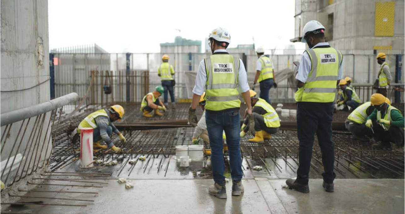
The new HSE handbook guides safe operations
