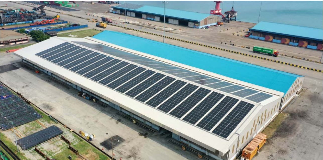
Solar PV panels installed at Kuantan Port
