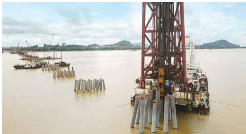
ICP Piles used in Batang Lupar Bridge Project, Sarawak
