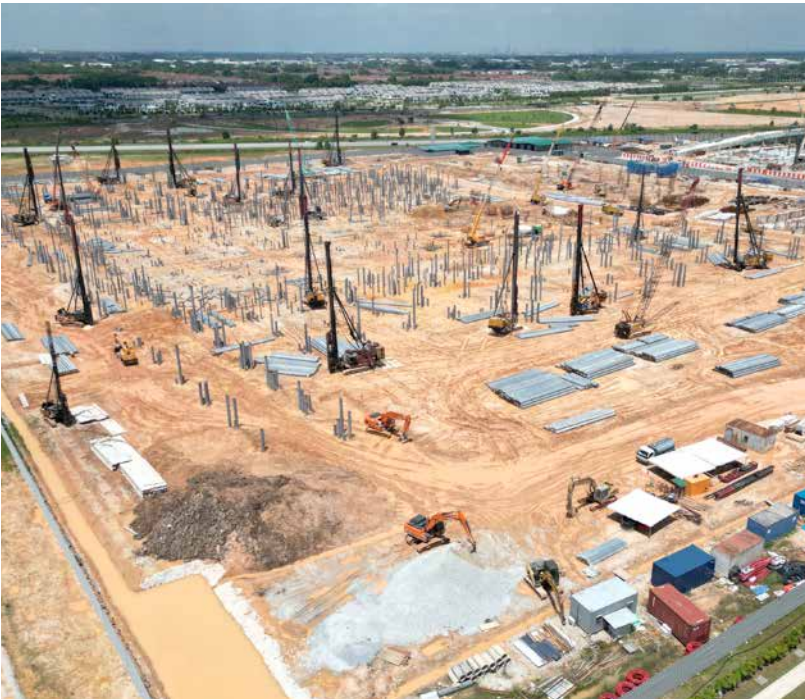
ICP piles at a project in Bukit Raja, Selangor
