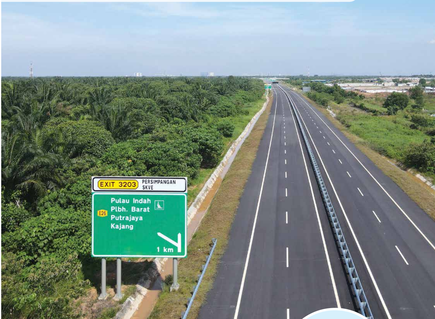
Section 2, West Coast Expressway
