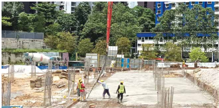
Concrete supply at the Pantai Sentral Park project, Kuala Lumpur
