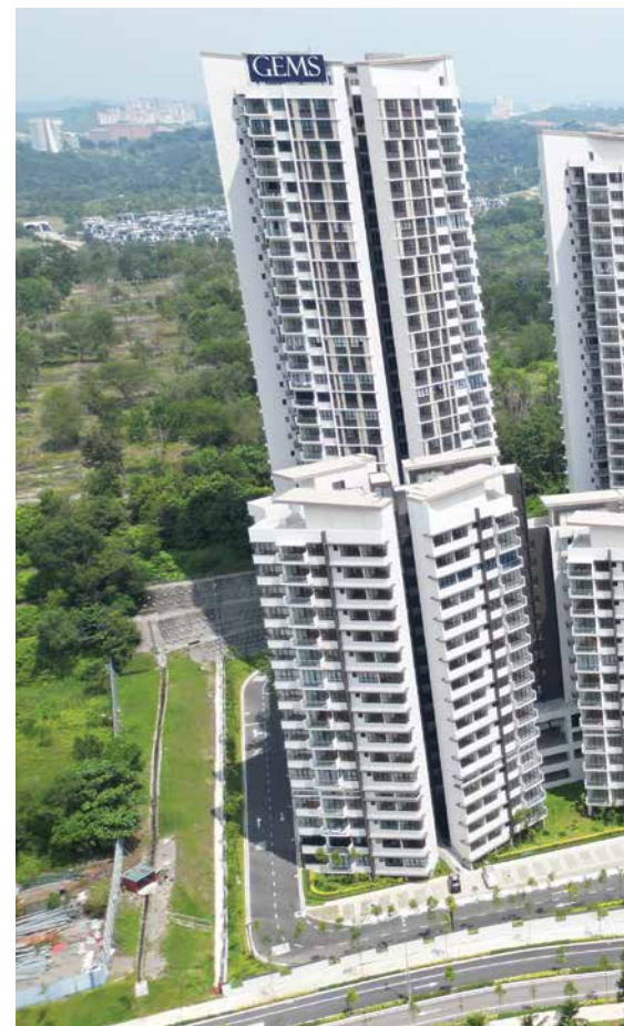
ICP piles used in the Gems Residences, Putrajaya
