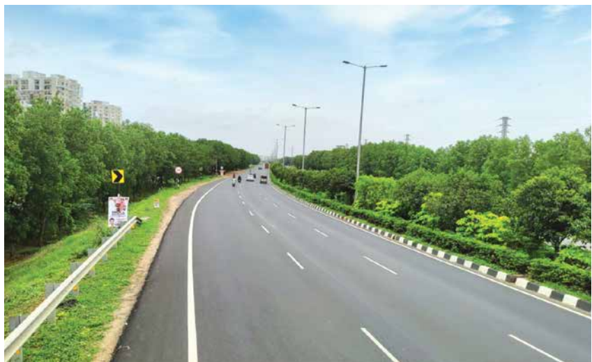
Completion of overlay at Chilikaluripet-Vijayawada Tollway, Andhra Pradesh, India
