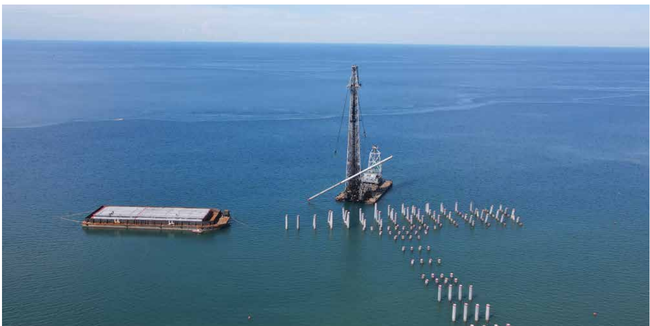
ICP piles at the Wanxiang Nickel Jetty, Morowali, Indonesia
