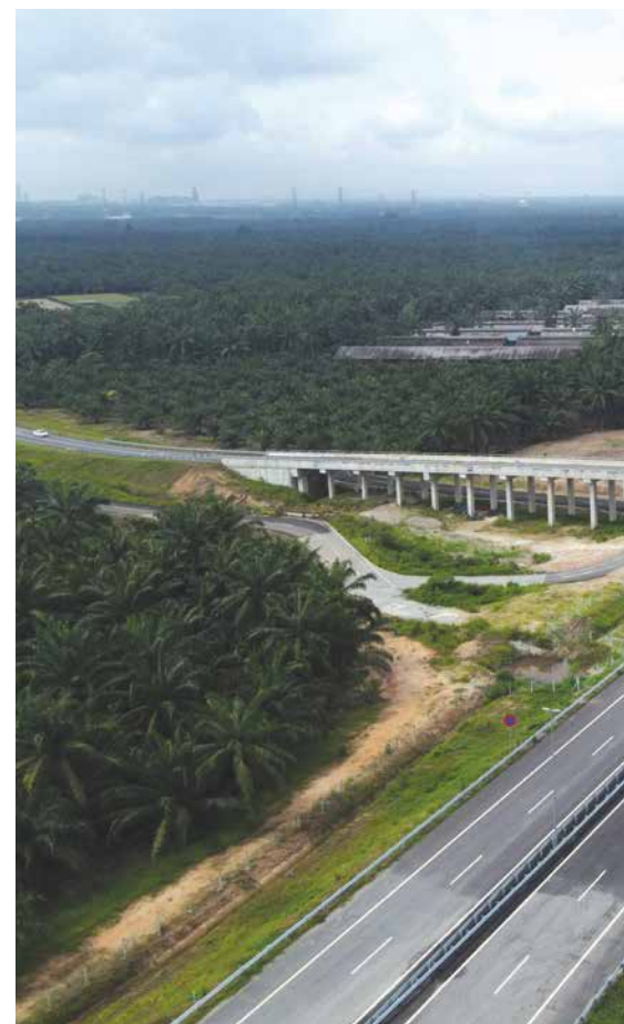
Section 1, West Coast Expressway
