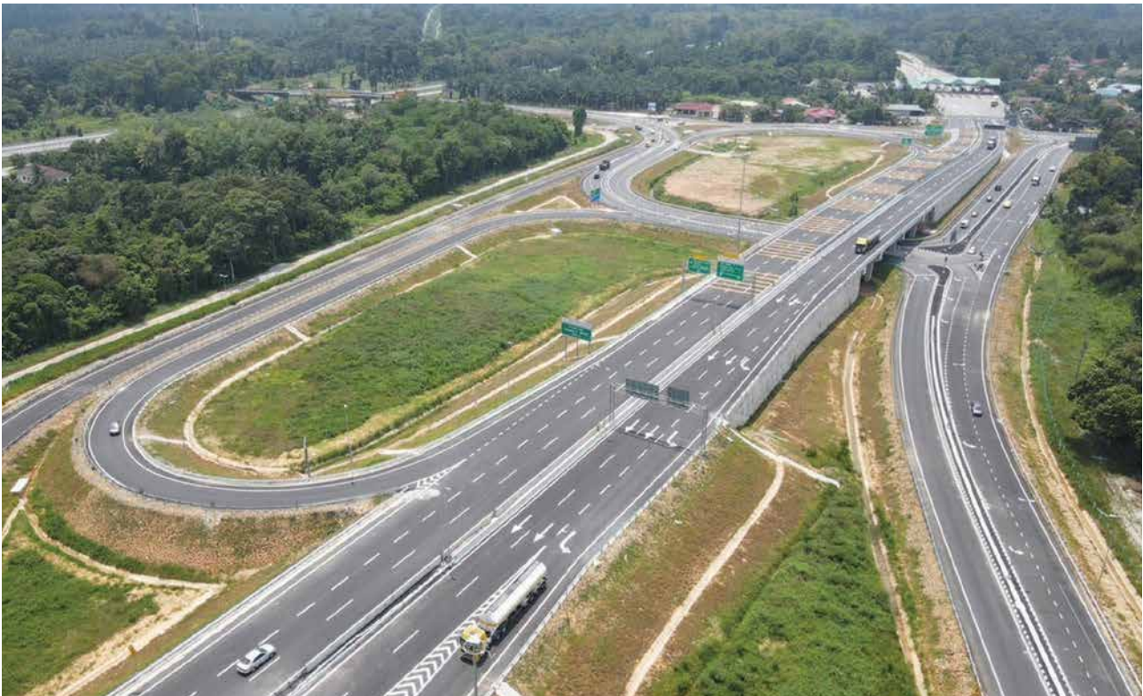
Section 11, West Coast Expressway
