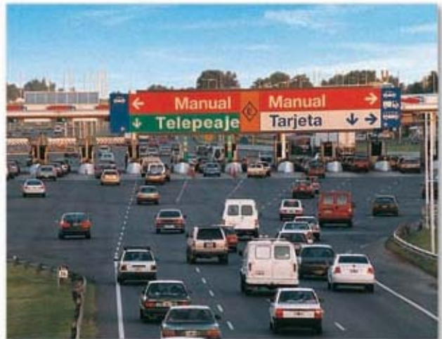
Western Access Tollway, Argentina
